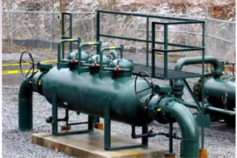
**A Field Proven CBM Filter.** *This revolutionary pipeline filter replaced a competitive unit (seen to the right) that required seven 4" x 36" elements. The new Sparks Series R100 filter with 3 elements has operated continuously for 6 months, without service, saving the CBM producer 75 hours of remote field maintenance and over \$20,000 in replacement filter elements.*
